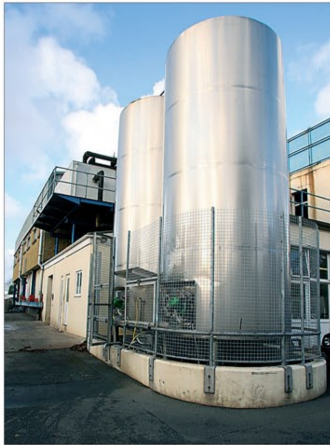
■ READY AND WAITING: These two 25,000-litre silos are filled with raw milk, ready for processing. (0506267)
